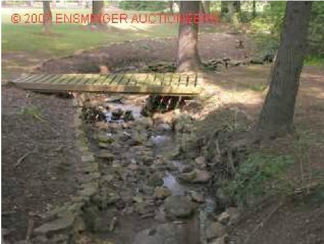
Bridge to the picnic area
