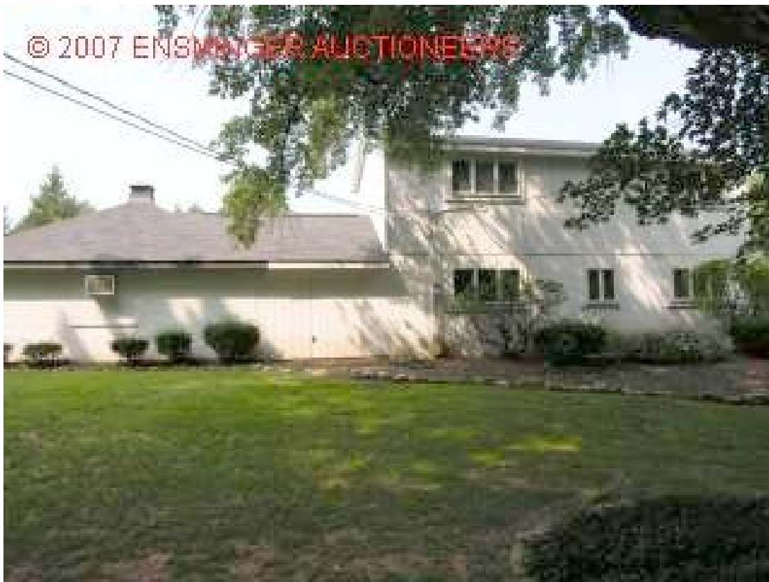
Left side of the house
