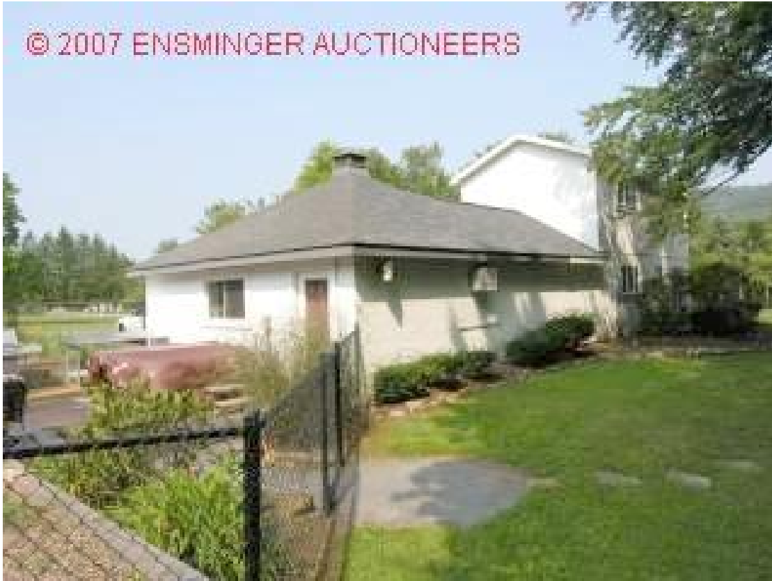
Rear view from the right rear corner
